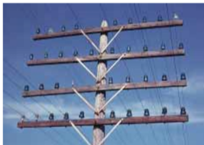
Electrical insulators on telephone poles are often made of glass because of its low electrical conductivity.
