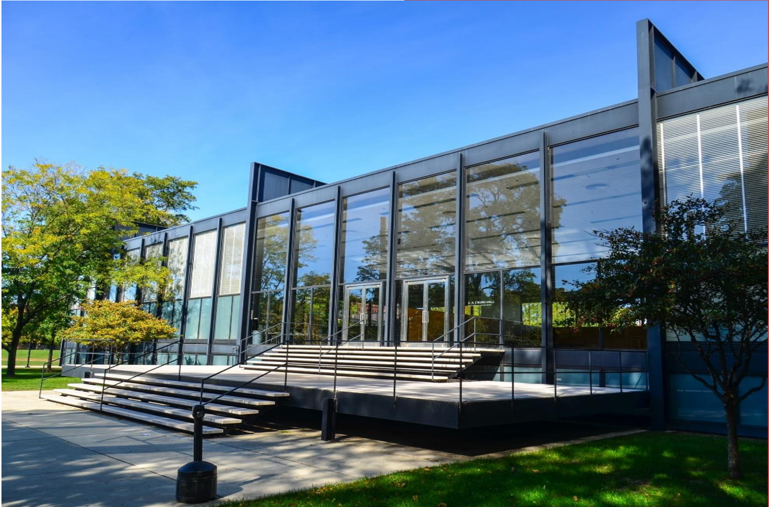
S. R. Crown Hall on the Illinois Institute of Technology campus. Designed by Ludwig Mies van der Rohe in 1956
