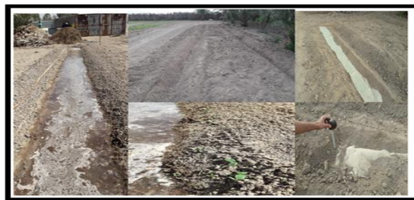
Figure 2: Installation of the membrane beneath the soil surface.
