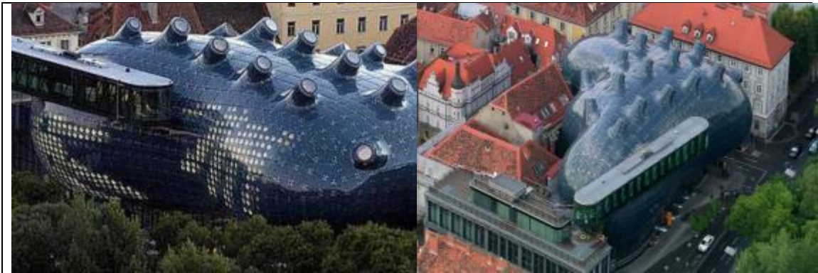
Fig.15 Kunsthaus Graz museum- Graz, Austria - designed by Peter Cook and Colin Fournier- The building's innovative complex double-curved geometric façade- an enormous biomorphic shell defined as "friends alien".
